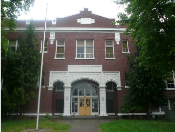
West elevation entry
