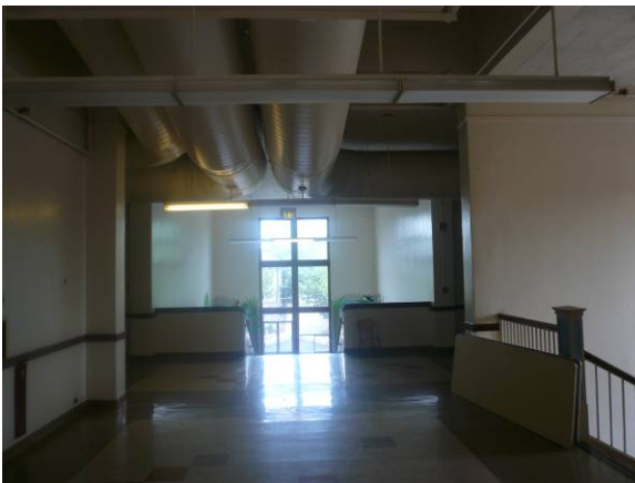
Corridor and exposed ductwork
