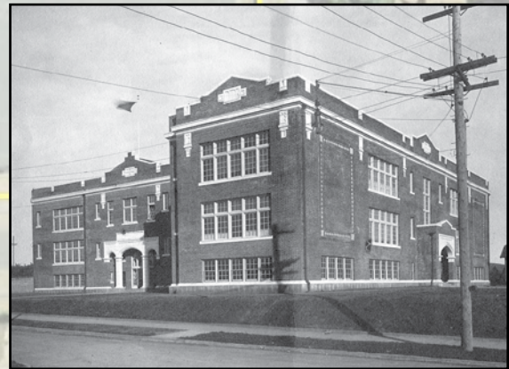
Mid-1910s photograph of Rose City Park School showing the newly completed unit 2 of the school. A matching unit 3 would be built on the opposite side of the courtyard soon afterward.
