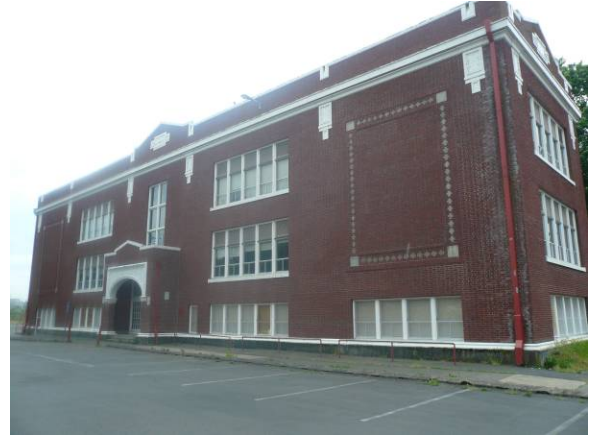
North elevation facing southeast
